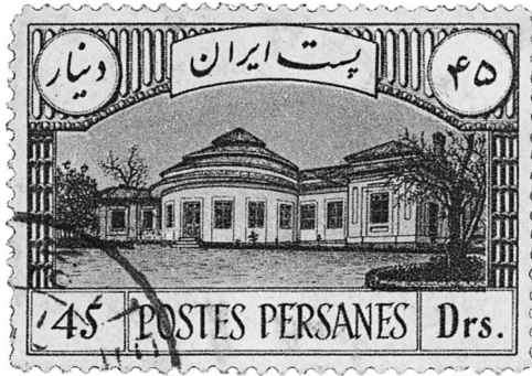
3.3 Sanatorium near Tehran
