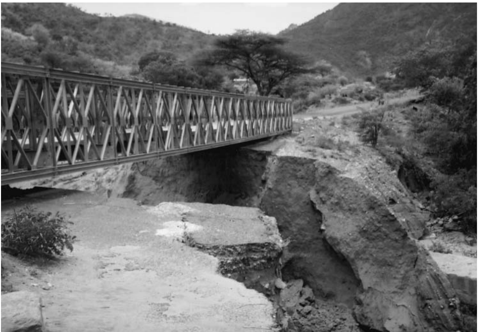
Plate 6.1 Temporary road bridge, Ortum, Kenya.
